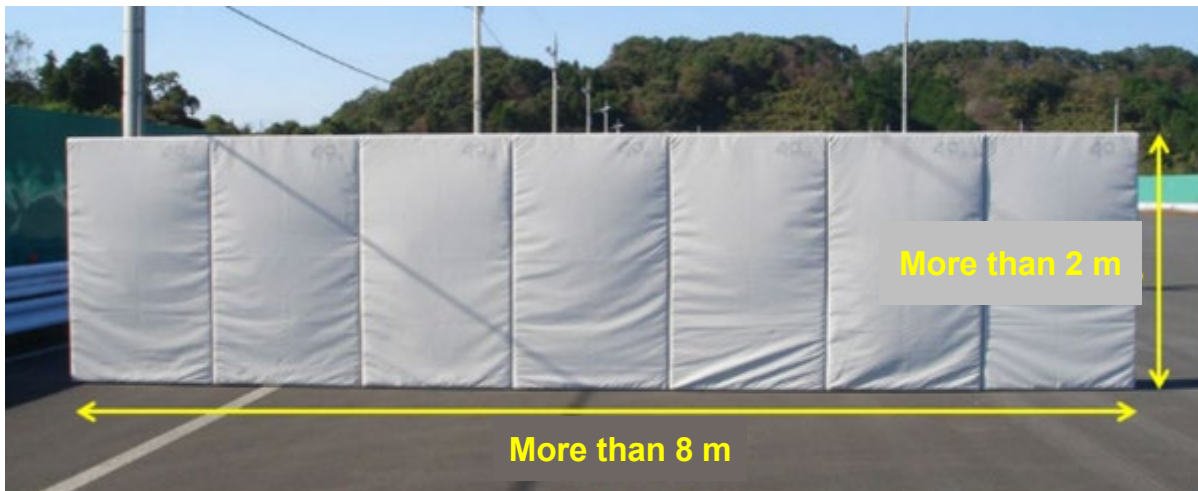
Attached Figure B. Appearance and required dimensions of shielding wall
